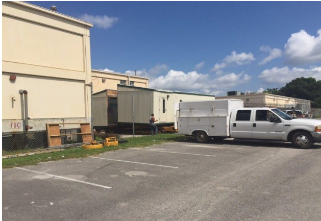
Portable Classroom Installation
